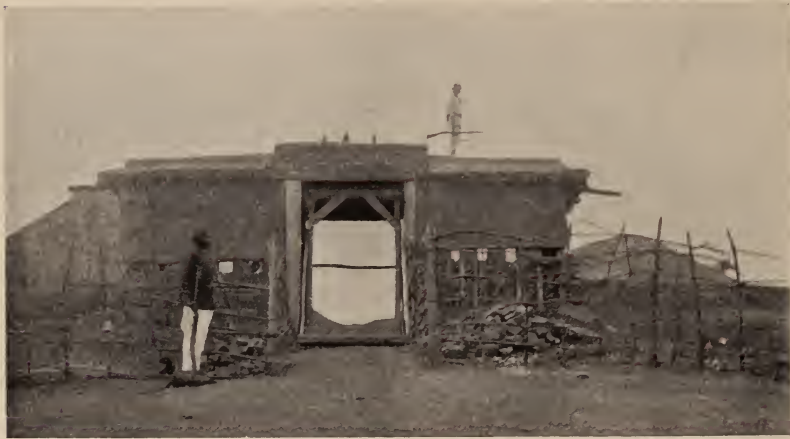
MAIN-ENTRANCE OF FORT KAMPALA.
